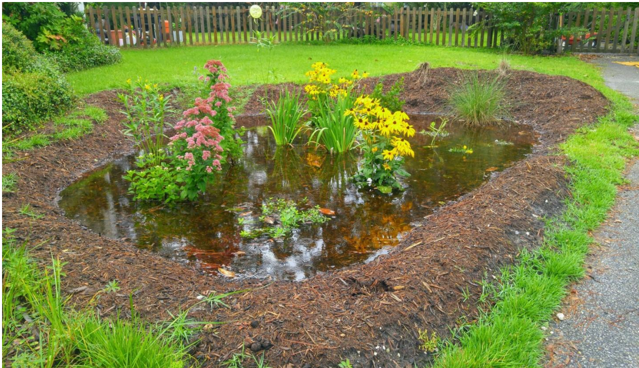
Example of a rain garden in a residential setting. Note: The rain garden depicted above is shown just after a rain event and should drain in less than 48 hours.
