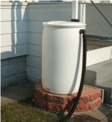
Notice sturdy base and overflow hose
